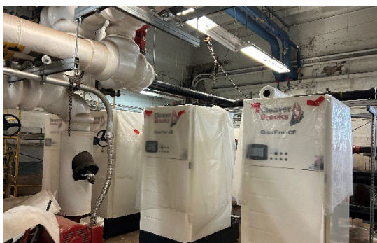
GP South New Hydronic Boilers
